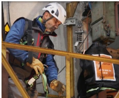
5/ Hook the 3 D-rings on the triangle with the descender connector,
